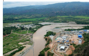
El Quimbo – HPP 400 MW (Under Construction) Com Operation 2016
