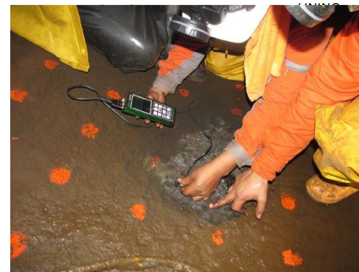
VERIFICATION BY UT
