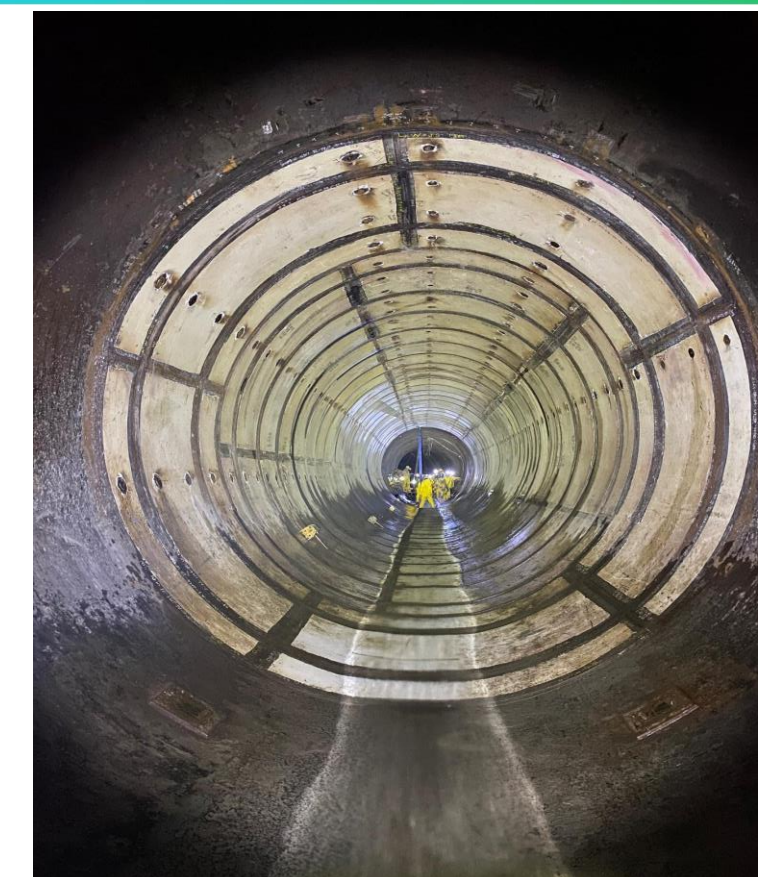
FINAL REPAIR IN PANDEO II –
