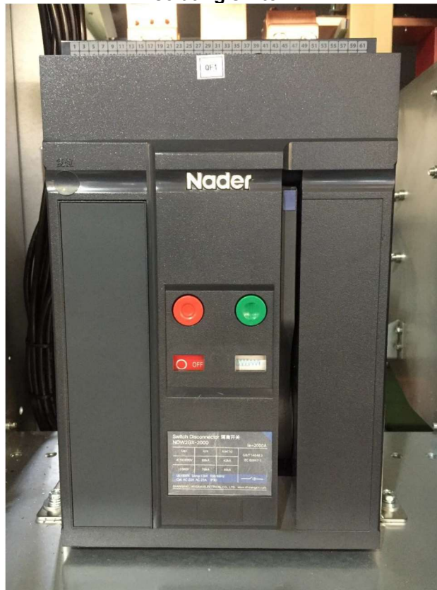
Isolating switch I
