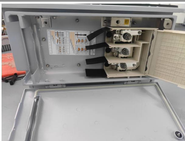
AC side terminal block
