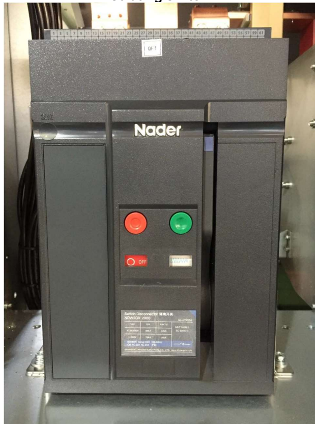
Isolating switch I
