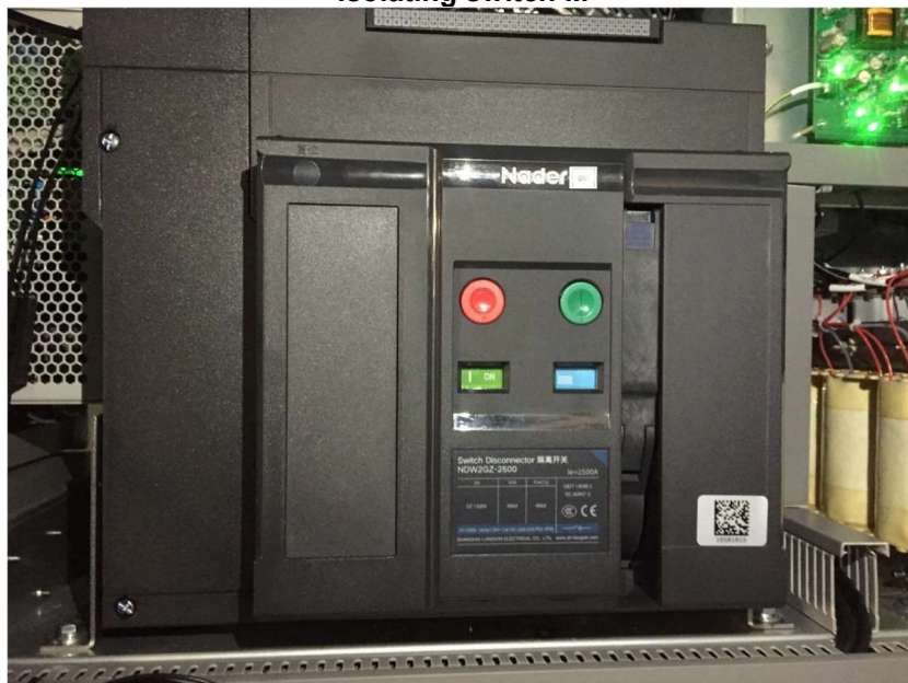
Isolating switch III
